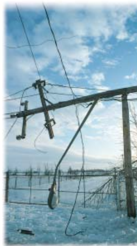
Figure 1.13 Downed power lines in Quebec during the 1998 ice storm
